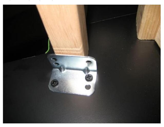
Here you can see there is exactly 1/4" of the L Shape sticking out beyond the bezel...perfect fit for the 1/4" plexi! (EDIT: Now using 1/4" glass).
